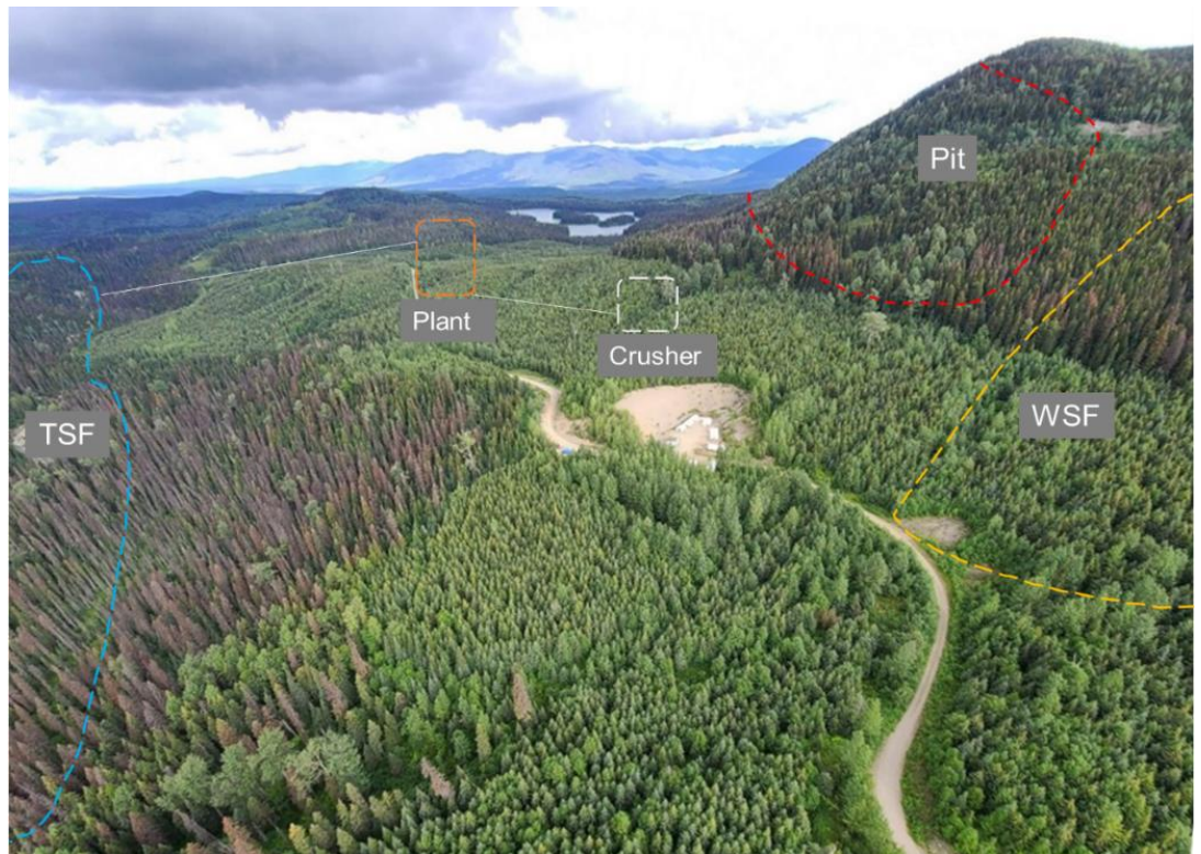
Fig 13 Wicheeda project, oblique view photo (viewing NE) – We have annotated the 2021 PEA site plan (below) on a best-efforts basis. On the right side of the photo is the deposit, part of a moderately-sloping mountain on the E side of the property. We note the waste storage facility (WSF) is situated in a hillside valley, making WSF design and construction simple from an engineering perspective. The crusher, plant, and TSF are all on gentle topography, allowing for relatively straightforward construction of supporting infrastructure.
