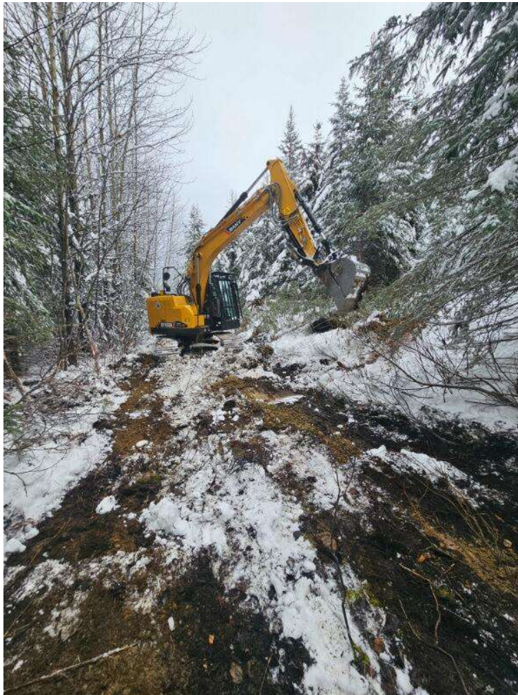
Image 3: Excavated Overburden Test Pits Underway in Tailings Study Area
