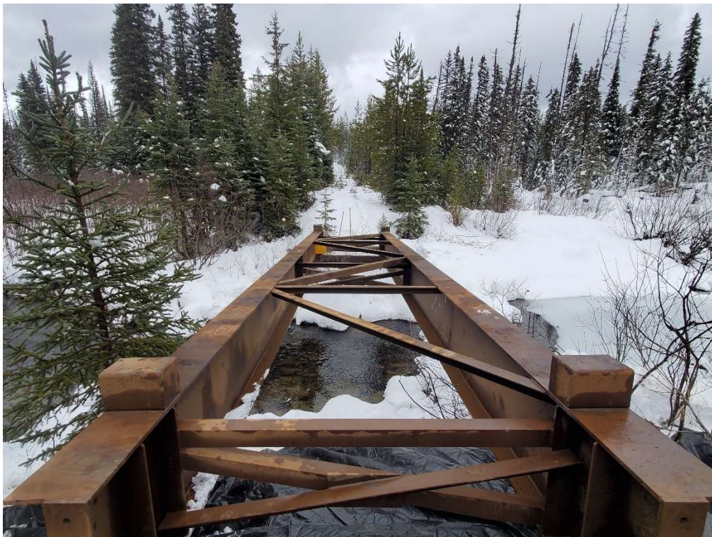
Image 2: Temporary Bridge Installation to Access Tailings Study Area
